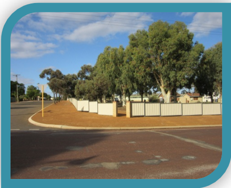
Caravan Park Fence Replacement
