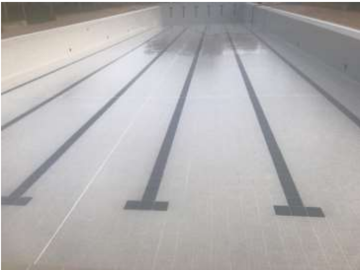
Corrigin Swimming Pool tile re-grouting
