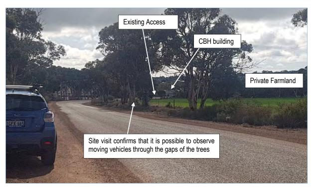
Figure 6: Sightline at Proposed Exit - Looking North
