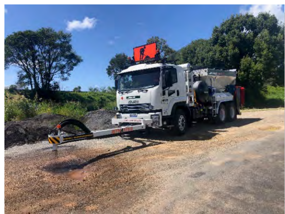
Example of Patching Boom position during operation.
