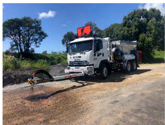
Example of Patching Boom position during operation.
