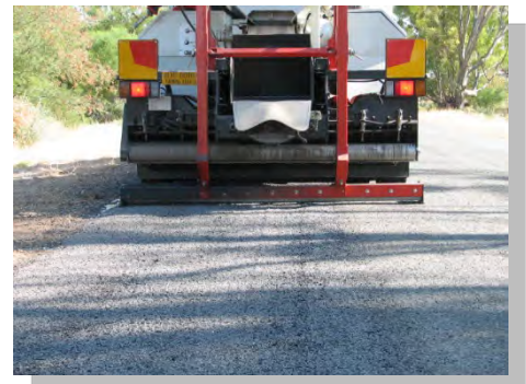
After wheel rutting repairs
