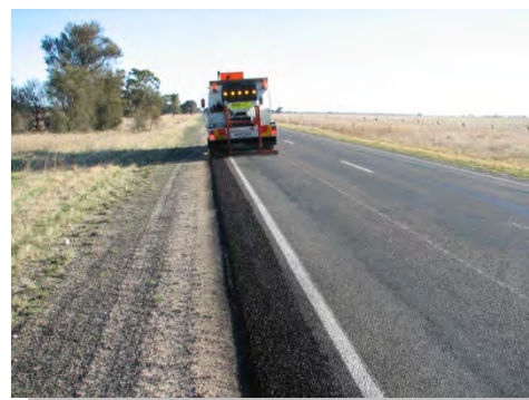
After shoulder sealing
