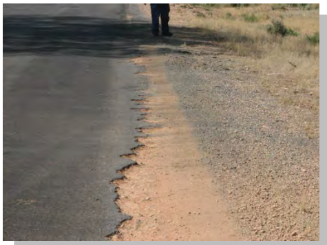
Before shoulder sealing
