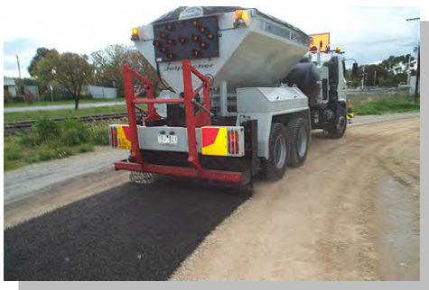
Spray sealing in progress
