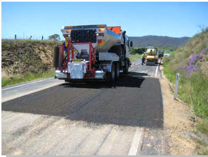
6m 3 control remote AUSROAD Jetmaster ® unit with aggregate spreader/spray bar, paving/edging attachment and road broom owned by Bega Valley Shire Council, NSW.
