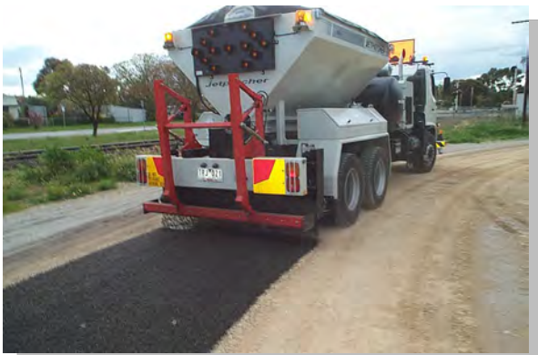
Spray sealing in progress
