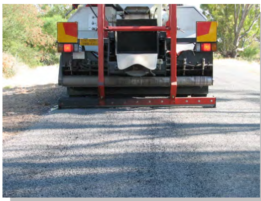
After wheel rutting repairs
