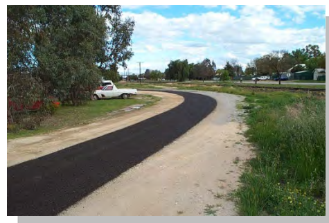
Completed Jetmaster® spray sealing
