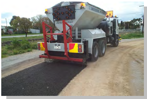
Spray sealing in progress
