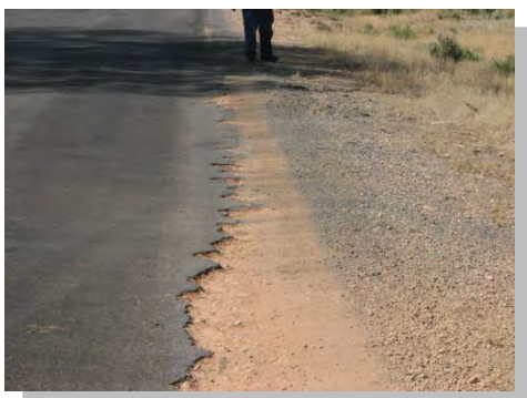
Before shoulder sealing
