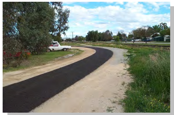
Completed spray sealing
