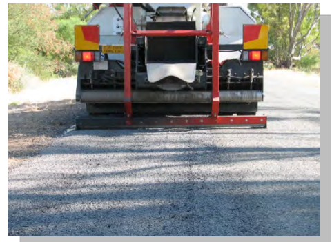
After wheel rutting repairs
