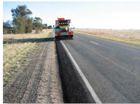
After shoulder sealing
