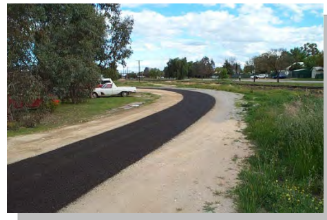
Completed Jetmaster® spray sealing
