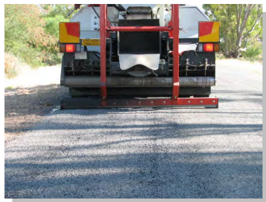
After wheel rutting repairs
