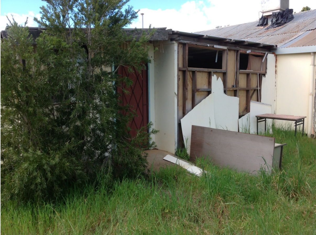
Rear of the premises at Lot 13, No. 10 Goyder Street, Corrigin (photo taken 13 August 2016)
