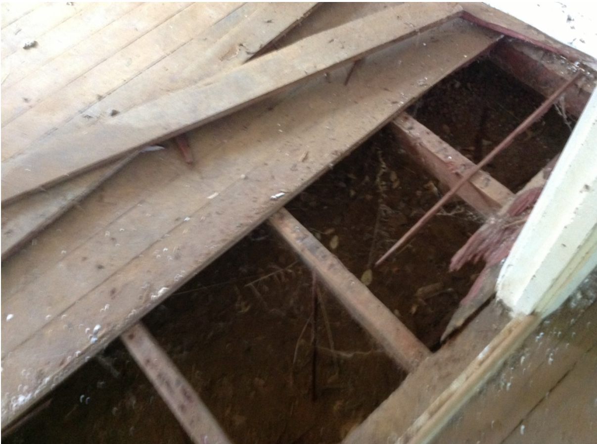
Damage to floor of the premises at Lot 13, No. 10 Goyder Street, Corrigin (photo taken 13 August 2016)
