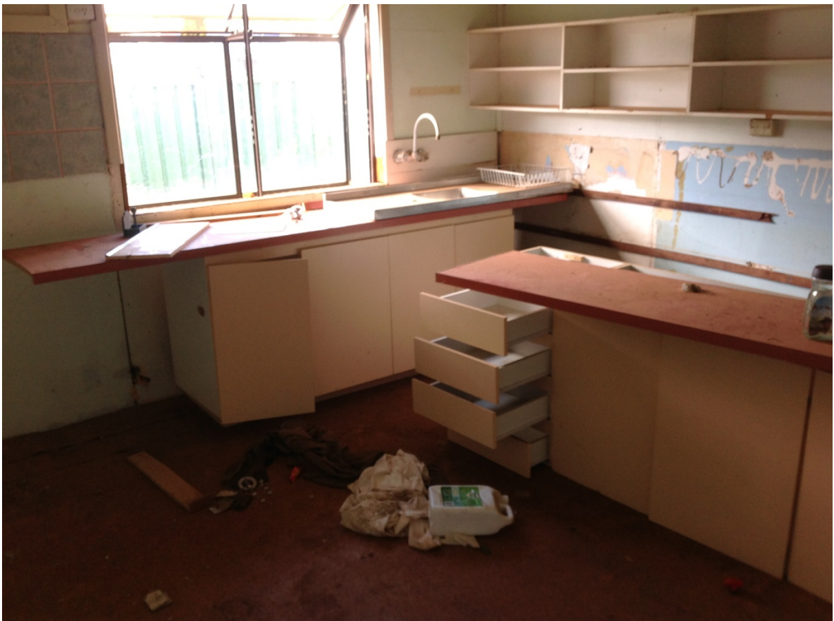
Kitchen of the premises at Lot 13, No. 10 Goyder Street, Corrigin (photo taken 13 August 2016)
