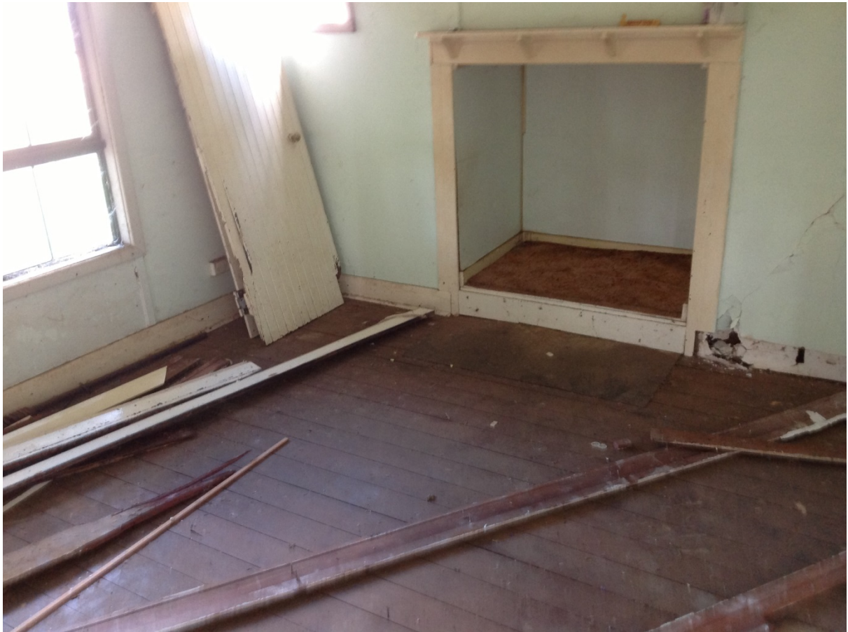
Internal damage to floor of the premises at Lot 13, No. 10 Goyder Street, Corrigin (photo taken 13 August 2016)
