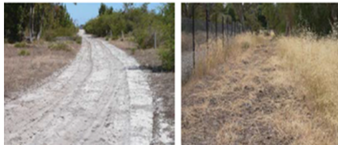
Acceptable Mineral Earth Firebreak
