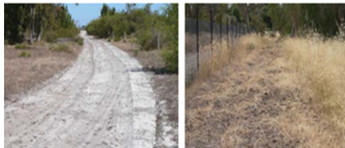
Acceptable Mineral Earth Firebreak
