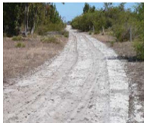
Acceptable mineral earth firebreak
