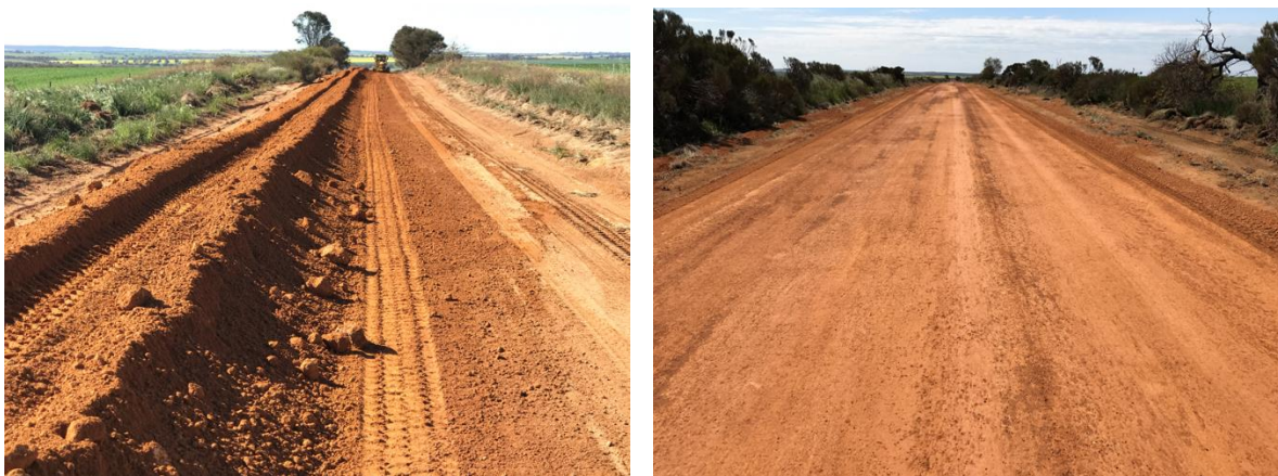
Lohoar Rd – example of gravel resheet
