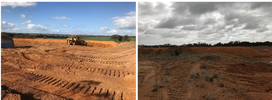
2 Dozers pushing up and stockpiling gravel at Hewetts Pit (Lohoar Rd SLK 2.81)
