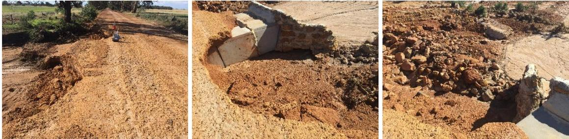
Dry Well Rd SLK 10.24 to 10.28 – example of severe damage (extensive scouring of embankment/shoulder, damage to culvert headwall and loss of rock armour protection)
